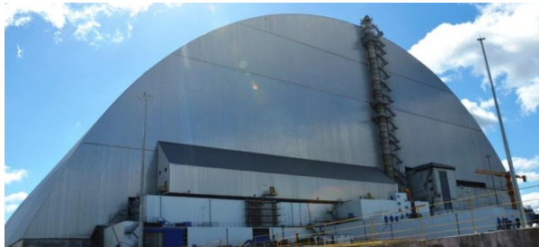
Fig. 1. Final view of NSC
