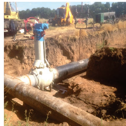
Fig. 4. DN 700 branch welded to the DN 1000 looping at the valve 8
