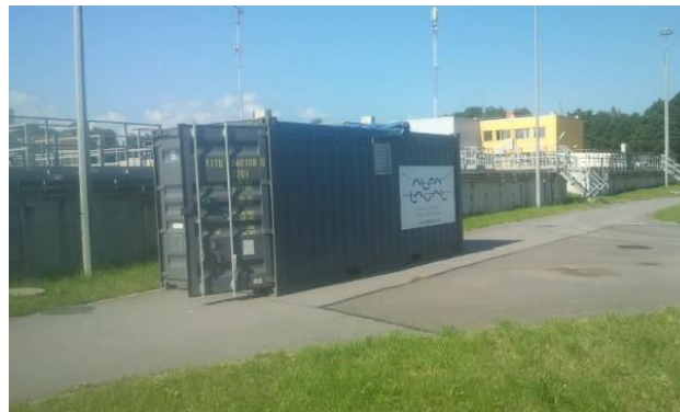
Fig. 1. General view of the membrane bioreactor “Alfa Laval” (Denmark)
