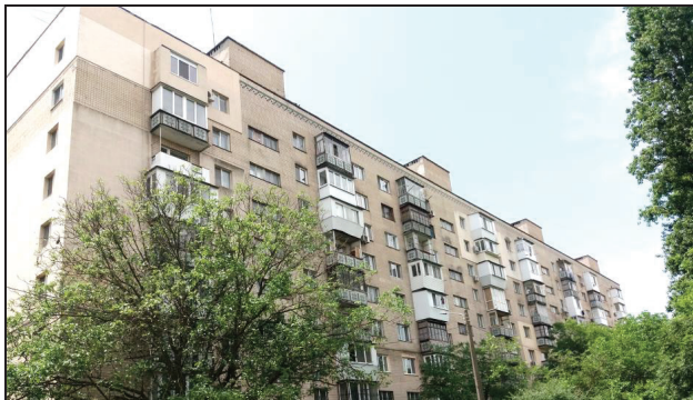
Fig. 1. General view of a 9-storied 144-apartment building
