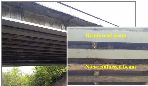
Fig. 1. Strengthening the reinforced concrete beams of a bridge with methyl methacrylate
