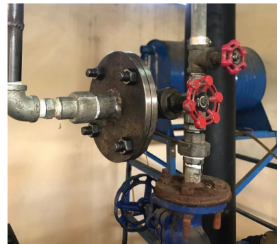
Fig. 3. Installation of the gasket on the flange in the boiler line
