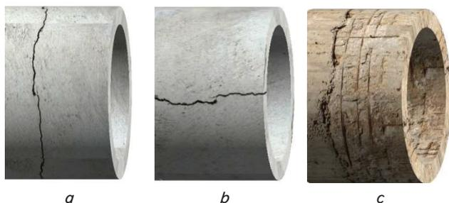
Fig. 1. Damage to pipes under operating conditions:
