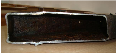
Fig. 10. Pipe fragment (140×60×3 mm) of the base of the body frame is affected by corrosion
