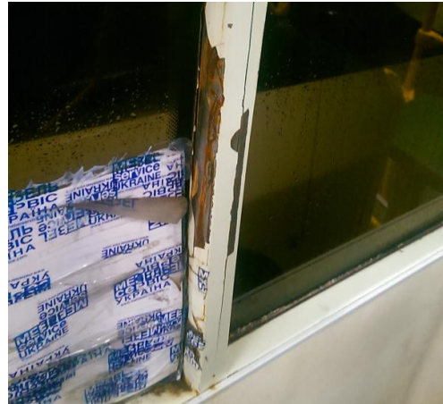
Fig. 8. Crack in the vertical rack of the cabin as a result of freezing of the accumulated moisture of the city bus «Ataman» A092H6
