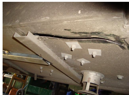
Fig. 9. Fatigue crack in the bottom of the compartment of the autonomous heater of the city bus «Ataman» A092N6
