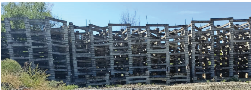
Fig. 6. Debris-flow control structure in the bed of Telavi river gorge
