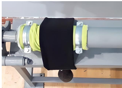
Fig. 2. Photo of the appearance of the installation
