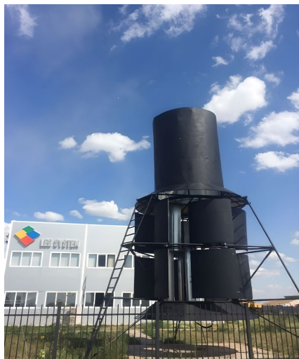
Fig. 8. Semi-industrial installation of a vortex wind turbine
