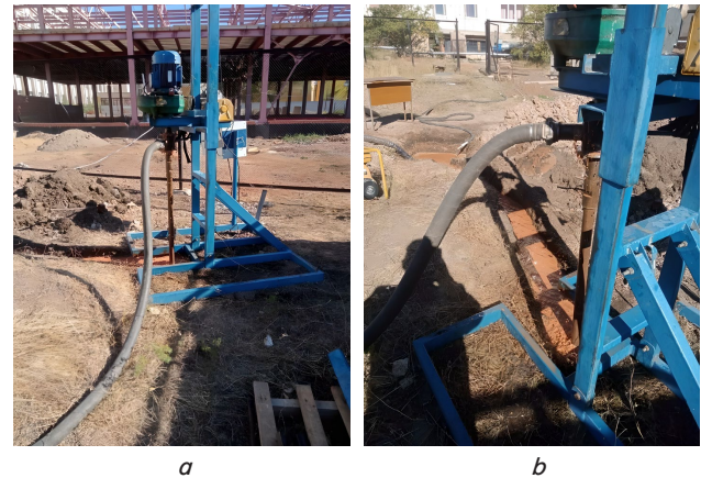
Fig. 5. Small drilling rig
