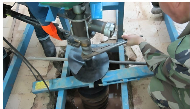
Fig. 3. Installation of suspended Equipment
