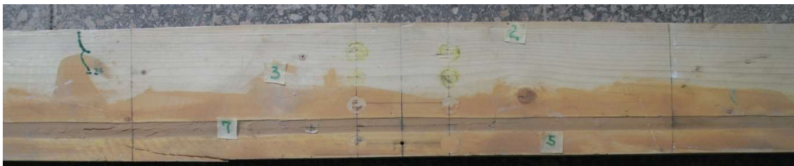
Fig. 9. Crack patterns of sample 1-Rd
