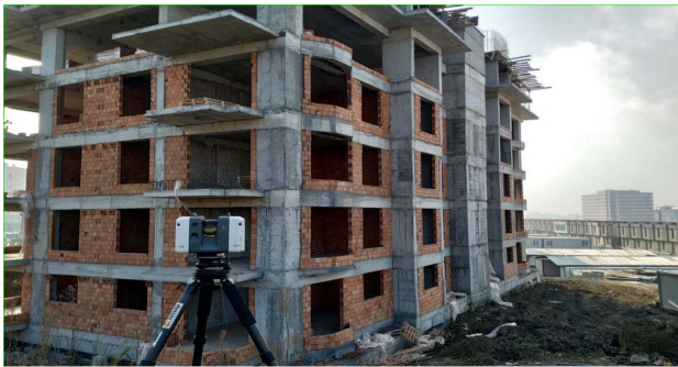
Fig. 4. The photograph was taken during laser scanning in the work area (prepared by authors)
