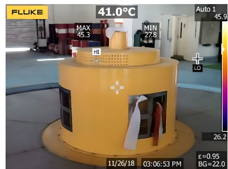
Fig. 10. Thermal data around the generator section
