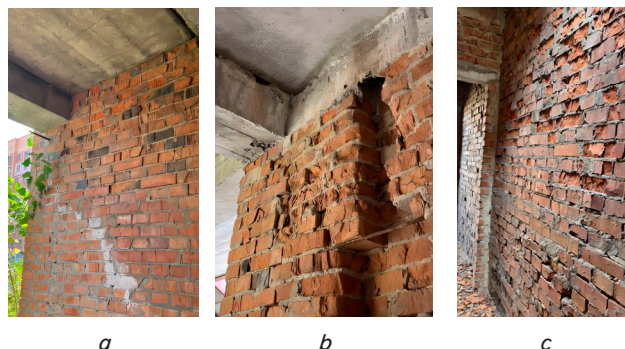
Fig. 2. Damage caused by frost heave to brick wall structures: a – damage to the internal partition; b – damage to the internal load-bearing wall; c – damage to the external load-bearing wall
