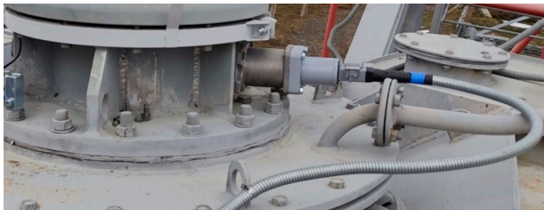
Fig. 11. Insulation test-tap adapter AIV-08, mounted on the bushing
