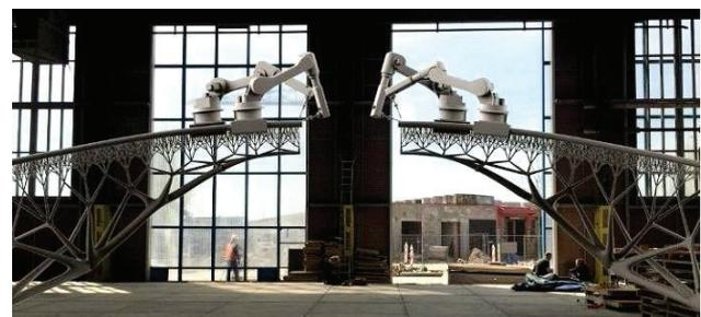
Fig. 13. The process of manufacturing a bridge using a welding 3D-printer [26]
