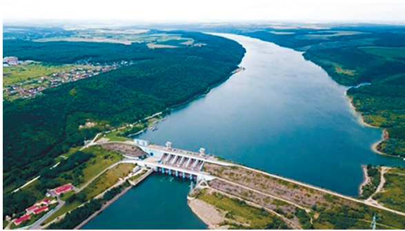
Fig. 2. General view of the Dnister HPP-1 and the reservoir [Online source: Official site of Dnister Water resources management].
