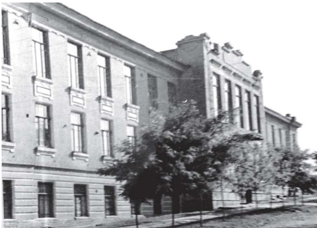
Oleksiivsky Hospital, where the Department of Pharmacology was located in the 20s of the XXth century
