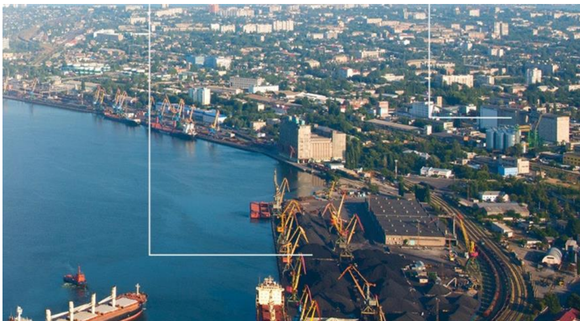
Fig. 3. Panorama of the results of the implementation of the infrastructure program of PJSC " Mykolaiv bread factory
