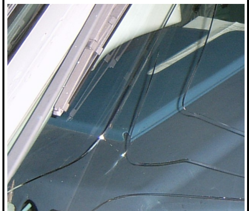
Fig. 2. Cracks in the cover glass
