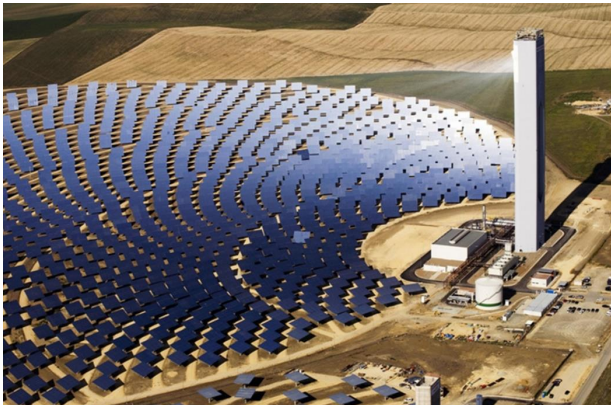
Fig. 2. Field of mirrors focusing solar radiation on the central receiver atop the tower of a solar tower power plant [12]
