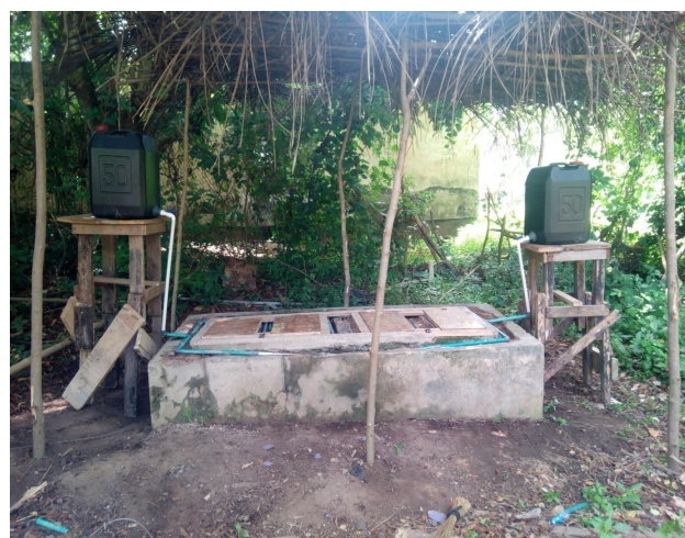
Fig. 1. Evaporative cooling chamber with water reservoir
