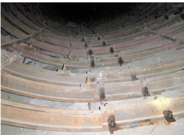
Fig. 12. Horseshoe-shaped reverse vault and anchors before concreting
