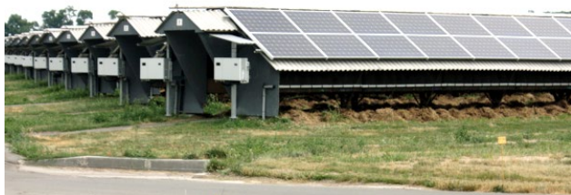
Fig. 1. Solar energy mini-complex for supplying individual workshops (production areas) of an industrial enterprise [15]
