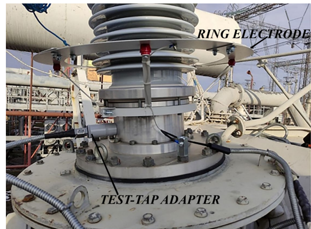
Fig. 5. Example of the ring electrode and the test-tap adapter installation
