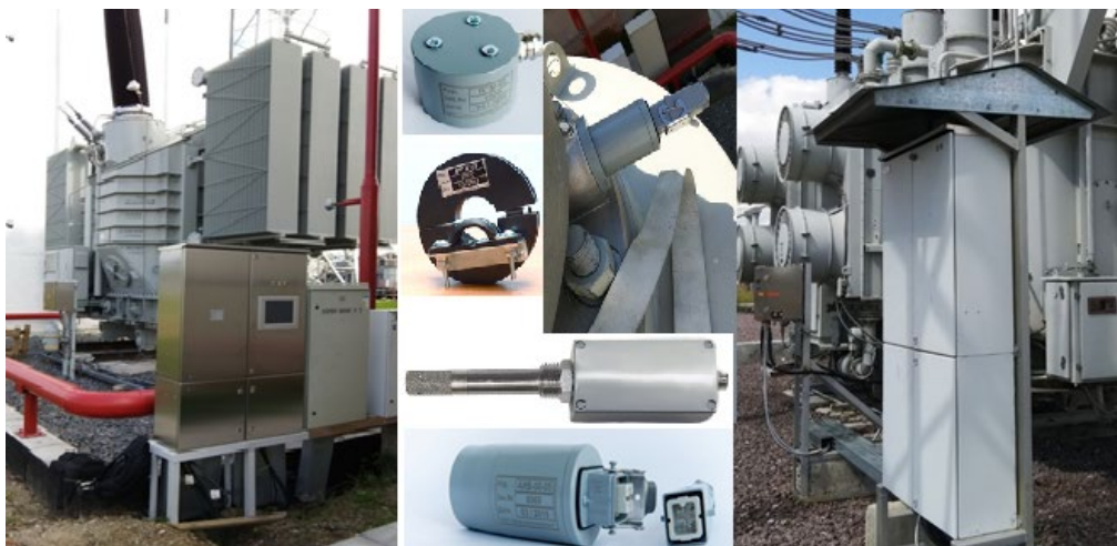
Fig. 1. Example of installation of the "full-range" OMS monitoring unit at the facility and some OMS's primary sensors
