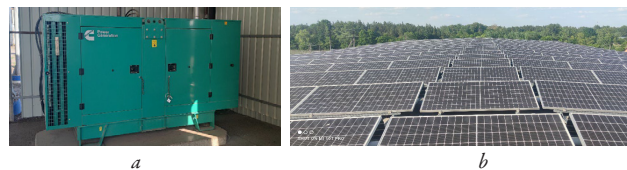
Fig. 4. General view of the elements that ensure the autonomy of the grain dryer, which are used in the process of corn grain drying at "Agrotechservice" LLC of the Poltava region: a – diesel generator; b – solar battery block
