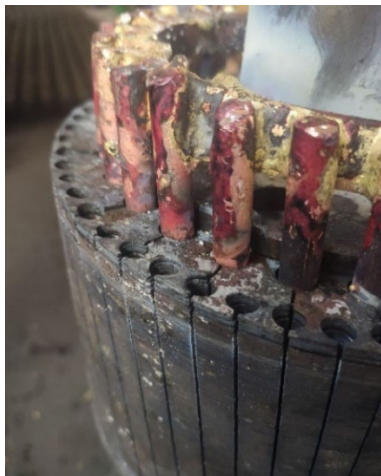
Fig. 2. Appearance of the rotor of an electric motor requiring replacement
