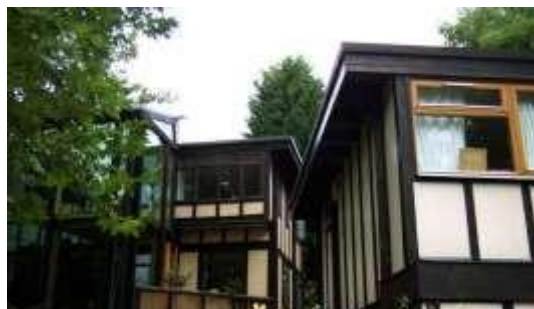
Figure 8. Walter's Project, 1976 Walter Segal http://architecture.about.com/od/periodsstyles/ig/House-Styles/The-Robie(House.htm)
